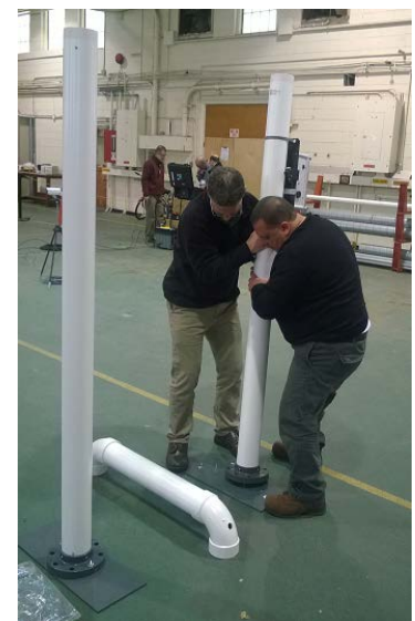
Figure 3-1 Evaluators assembling a PRPM
